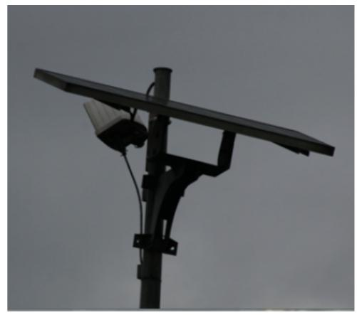
Traffic Sensor Powered by Solar Energy
