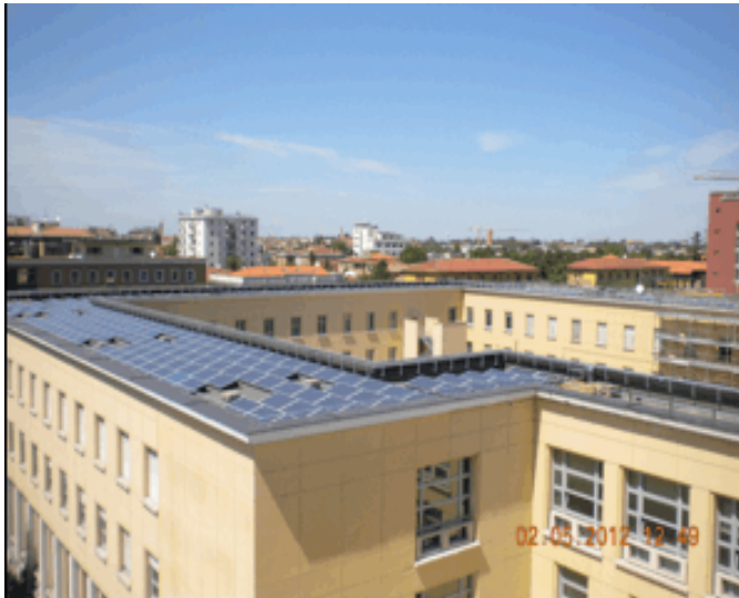
Photovoltaic installation on the roof of Palmezzano school
