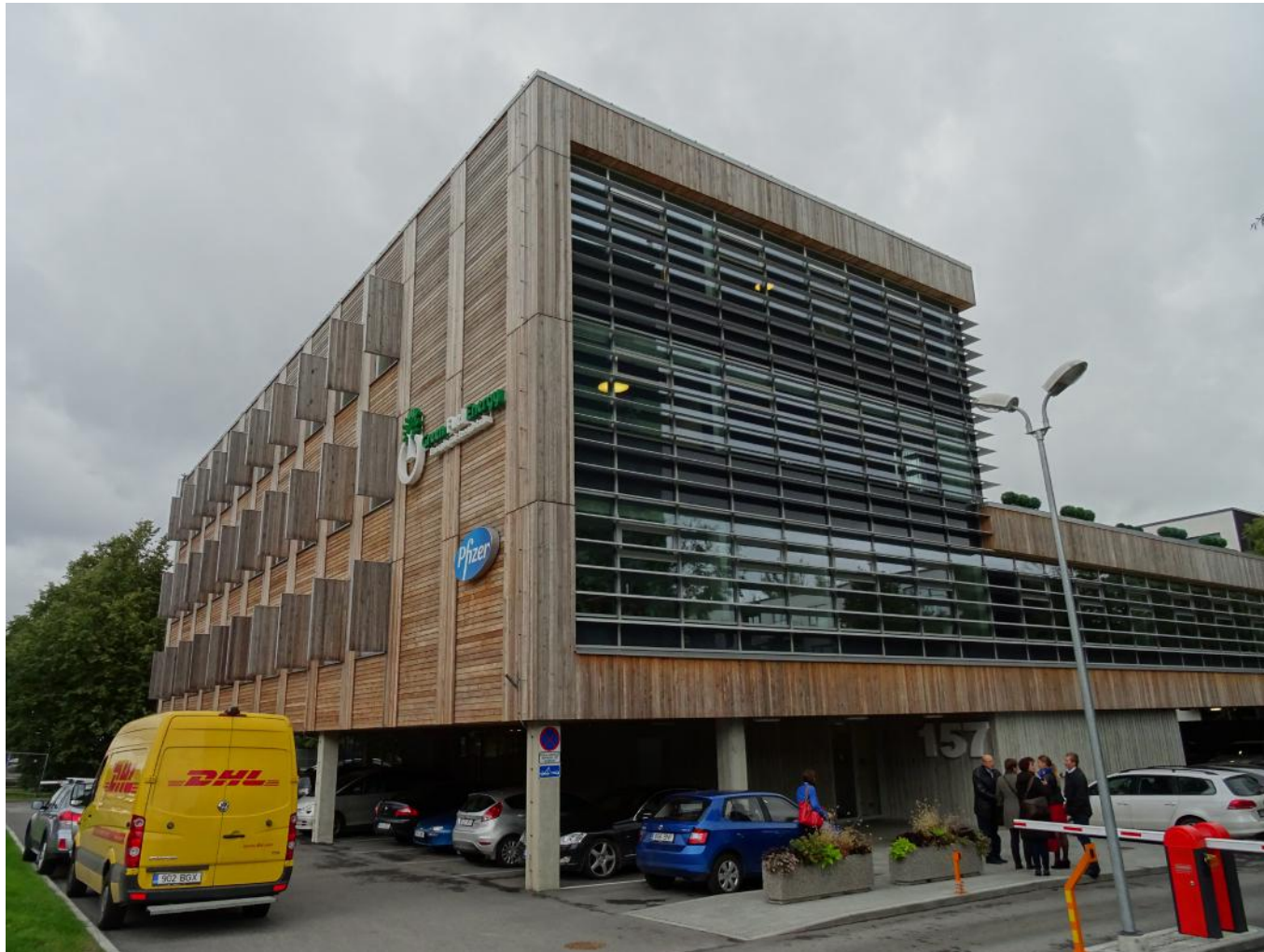
Example of energy efficient building, using a heat pump with the source integrated in the foundation and PV panels.
